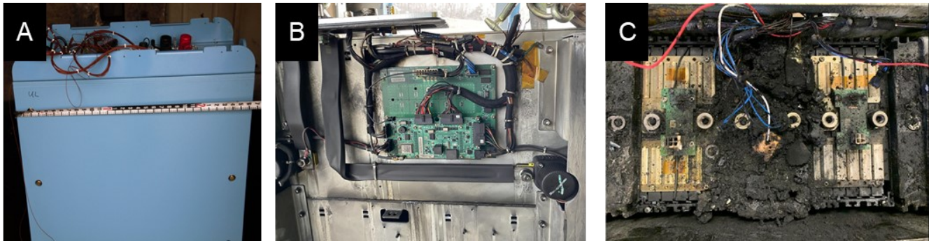
Figure 3. An ElectroVaya 24V battery pack shown after fire propagating testing in which a single cell was forcibly ignited, depicting (A) unscathed battery enclosure and external connections, (B) intact battery management system, and (C) no fire propagation between adjacent modules.
